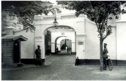
Photo : Front Gate of Benteng Ujungpandang, Early 20 th Century Source : BPCB Sulsel 2017
